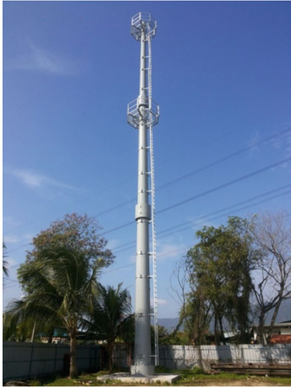
Fig. 1 UHPFC communication tower located in Malaysia
