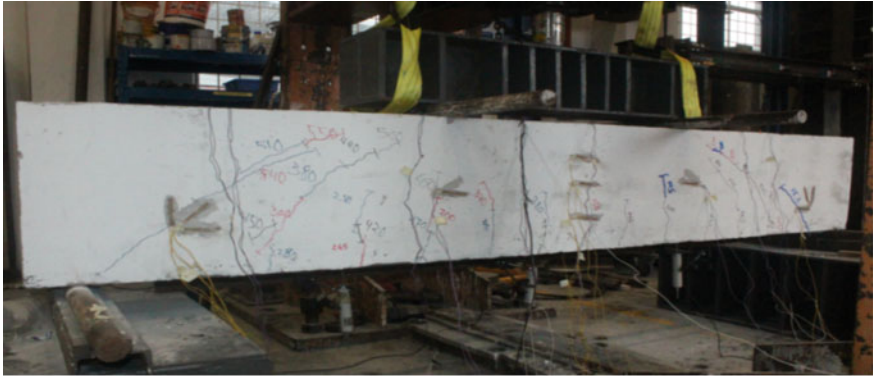
(a) RC crack pattern front view
