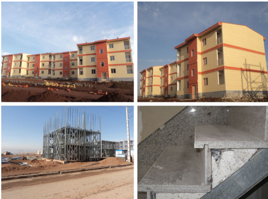
Fig. 3 Actual model of CFS in Pardis of Tehran
