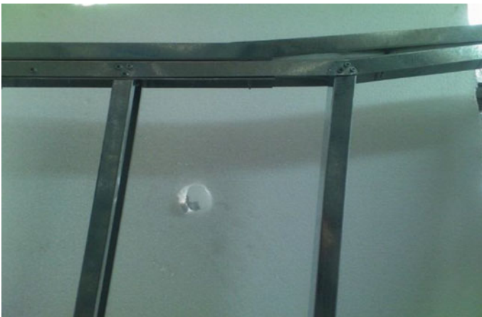
Fig. 9 Local buckling of connection in first specimen
