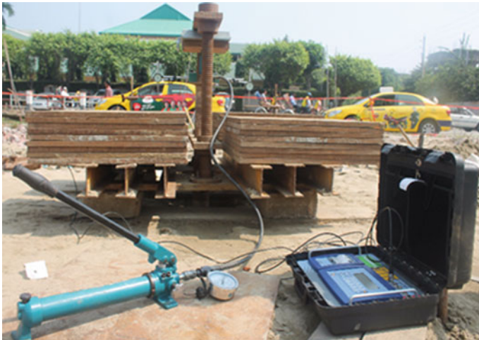
Fig. 2 Screw plate load test setup
