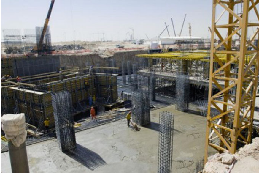
Fig. 3 KAFD construction work in progress
