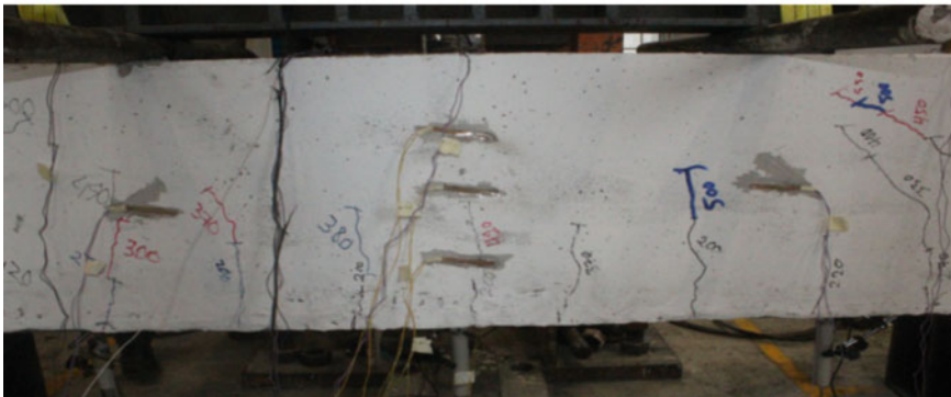
(c) RC crack left view
