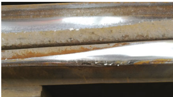
Fig. 1 Spalling defects of turnout
