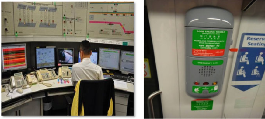
Fig. 2 Video monitor and emergency talking devices in FAO
