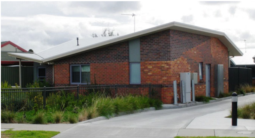
Fig. 1 Picture of one of the low-energy houses in 2012. Source Trivess Moore
