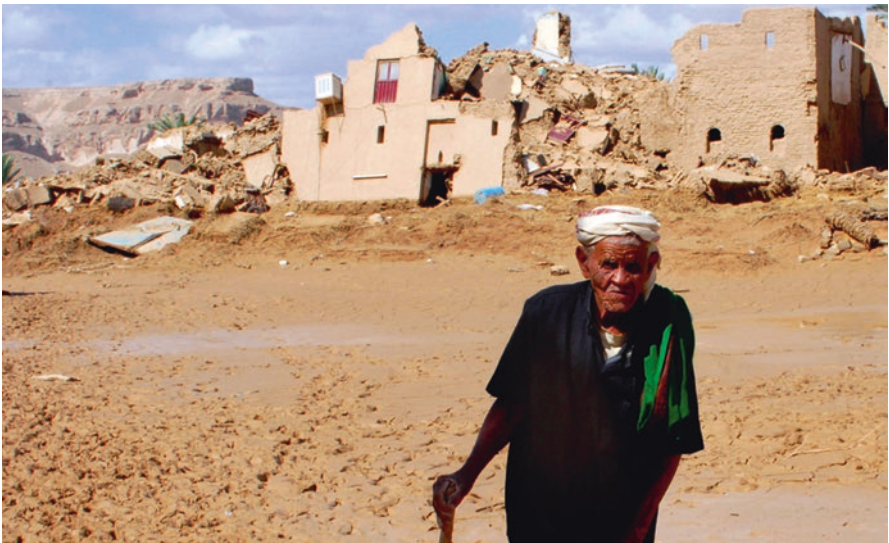
Fig. 3.13 Ninety-year-old Yemeni man walks in front of his family's collapsed houses in Wadi Hadhramaut on October 27, 2008 ( Source: The authors)
