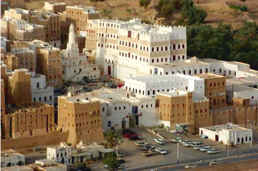
Fig. 3.4 Part of Shibam city in Hadhramaut showing different kinds of mud architecture buildings (Source: The authors)
