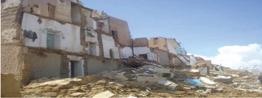
Fig. 3.1 A town to the east of Tarim city in Wadi Hadhramaut was destroyed, losing approximately 100 buildings during 2008 flash floods in Hadhramaut ( Source: The authors )
