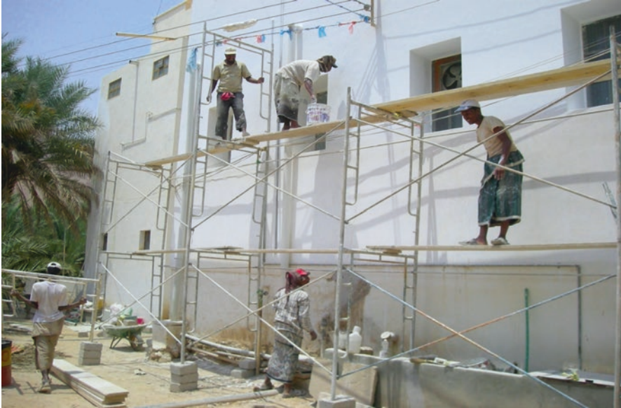
Fig. 3.14 Using lime in plastering the exterior of the houses at the most areas in Wadi Hadhramaut by rich families ( Source: The authors )
