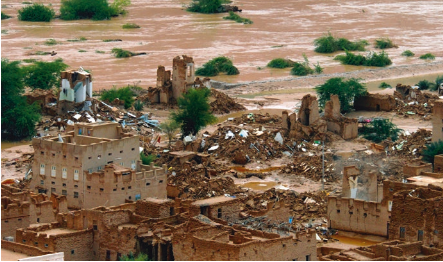
Fig. 3.15 Collapsed of mud buildings are seen surrounded by flash flood in a town in the Yemeni province of Hadhramaut on October 2008 ( Source: The authors )
