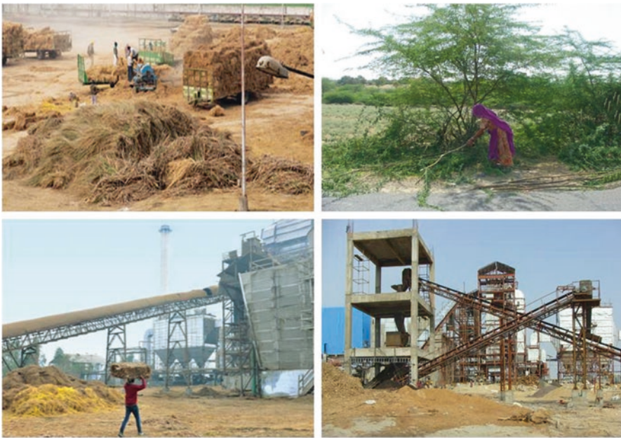
Fig. 31.1 Top left, utilization of rice straw is possible as animal feed and industrial use, including power generation; bottom left, view of a 12 MW biomass power plant in India that may utilize rice straw and other crop residues; top right, harvesting of Prosopis juliflora wood for domestic fuel use and also to feed biomass power plants in Rajasthan; bottom right, full view of a 10 MW biomass power plant (Transtech Green Power Limited) based on Prosopis juliflora and other wood wastes in Sanchore district (Rajasthan)
