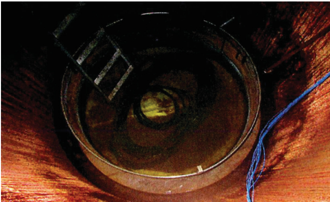
Fig. 8. Cable sample state after immersion in extreme alkaline solution
