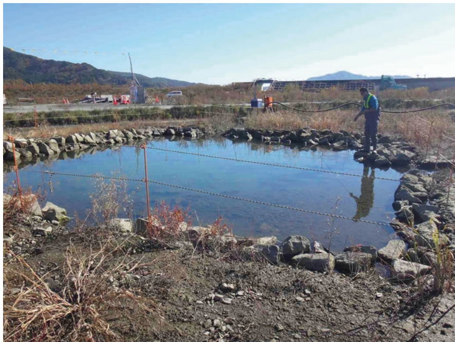
Fig. 13.10 Pond with spring water that was newly artificially created due to the mitigation of aquatic life conservation (Nov. 5, 2015). The blue and orange boxes beyond the pond are the pumping equipment. The depth was also artificially excavated in a rope enclosed
