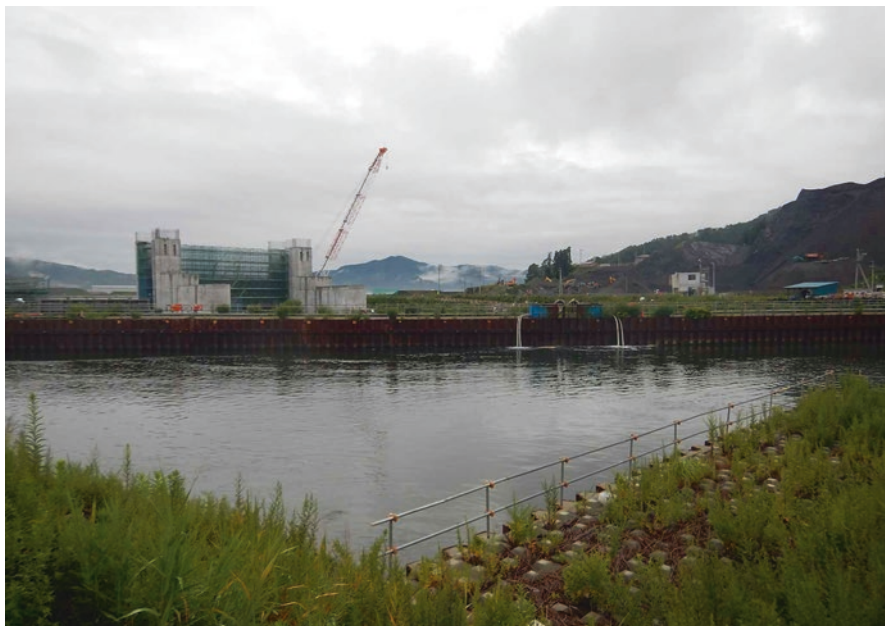
Fig. 13.7 Drainages from construction site of floodgate in the mouth of Kotsuchi River (Jul. 29, 2017)
