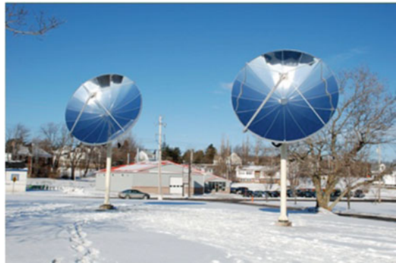
Fig. 5 Installed parabolic dish collector Image Courtesy: Solartron energy systems
