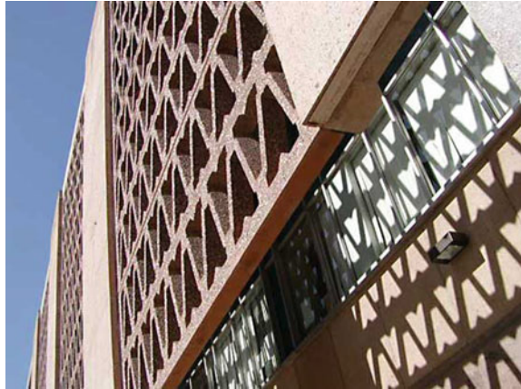
Fig. 5 Concrete brise soleil ( https://www.britannica.com/technology/brise-soleil )
