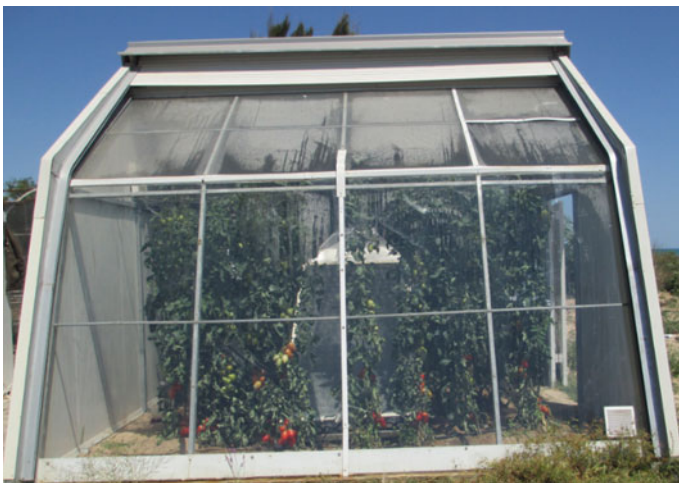
Fig. 2 External view of the greenhouse
