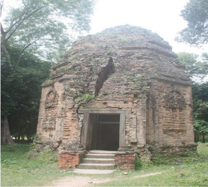
Fig. 14.2 Title: The N 7 Temple in Ishanapura (Cambodia). There are ten octagonal temples in Ishanapura. In the north group of temples only N 7 is octagonal. These temples are octagonal from the base to pinnacle. Top to bottom octagonal brick temples in India are not known. These temples are called flying palaces since on the outer side walls of the temple, palaces are shown being carried by sculpted winged animals. Source: Author
