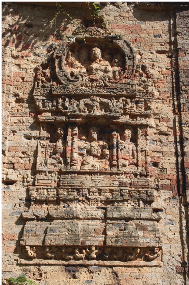
Fig. 19.6 'Flying Palace' on the exterior wall of an octagonal brick temple in the Southern group at Sambor Prei Kuk, Cambodia. Source: Author
