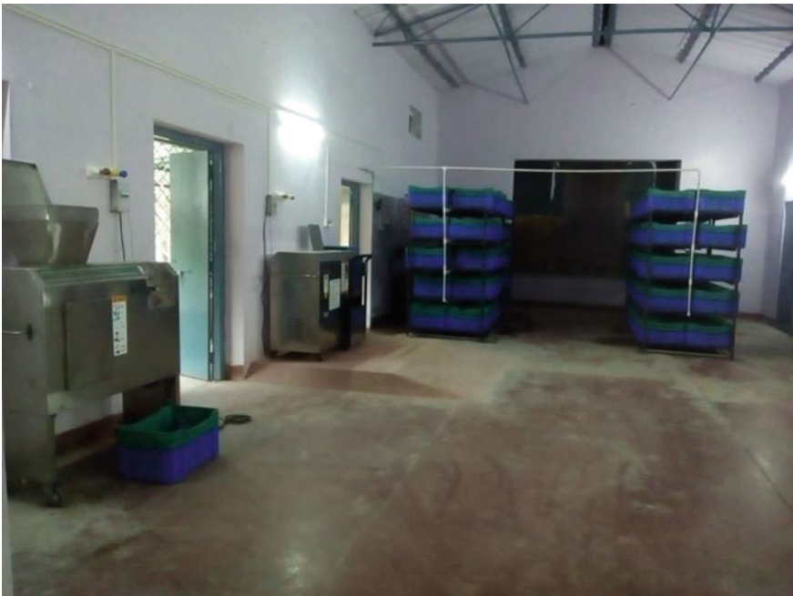
Photo 6 Newly installed mechanical composter
