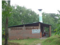
Photo 6: Waste Management Plant in KUET
