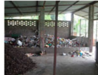
Photo 7: Degradable and non-degradable wastes in SWM plant
