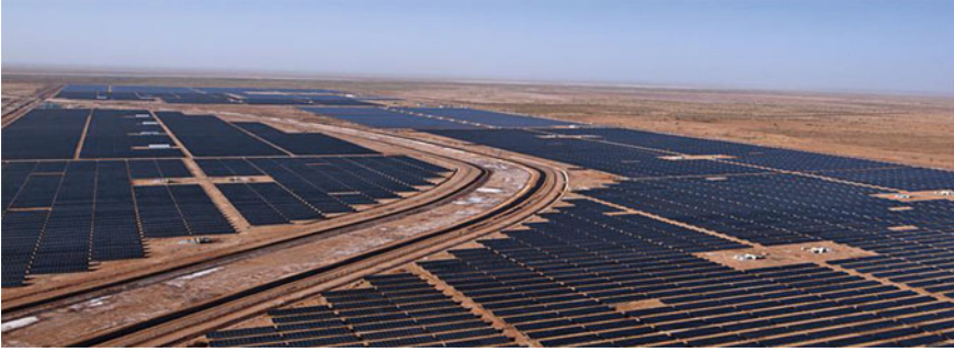
Fig. 2.4 A photograph of Gujrat solar park [7]
