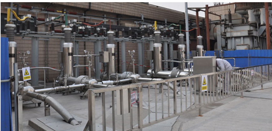
Fig. 3.16 35 kV 2000 A CD HTS cable terminal
