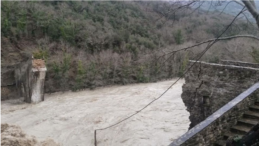
Fig. 6 The remains of the bridge after destruction ( http://epirusgate.blogspot.gr/2015/02/blog-post_32.html )
