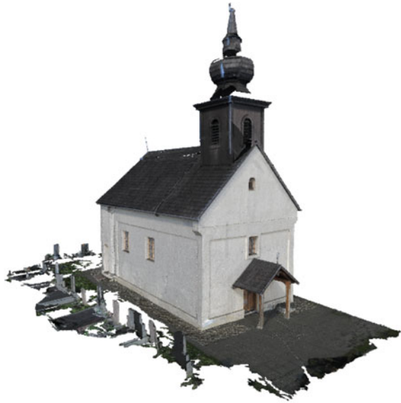
Fig. 9 Exterior model of the Kolozsnéma church. Point cloud colored from only 21 images using the vertex-based method
