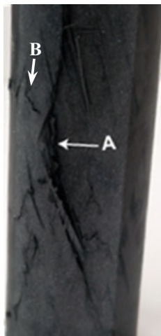
Fig. 10 Postmortem images of uncoated tubes showing a through-thickness axial cracks and b smaller circumferential cracks
