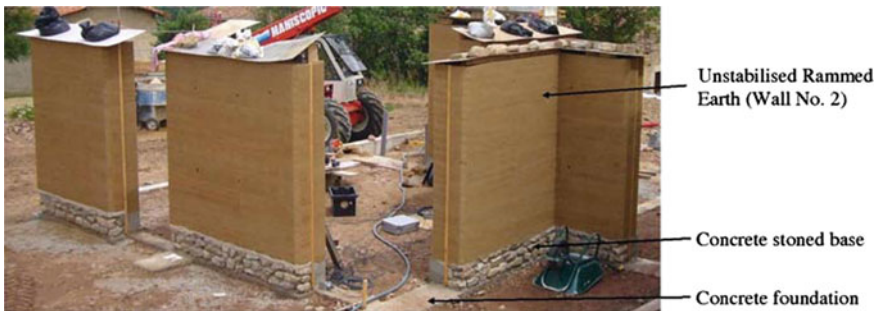
Fig. 6 In situ RE walls
