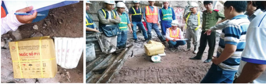
Fig. 4 Checking 102 kg of explosive type P113
