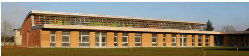
Fig. 1 A school with walls in RE constructed recently in France, Architect: V. Rigassi
