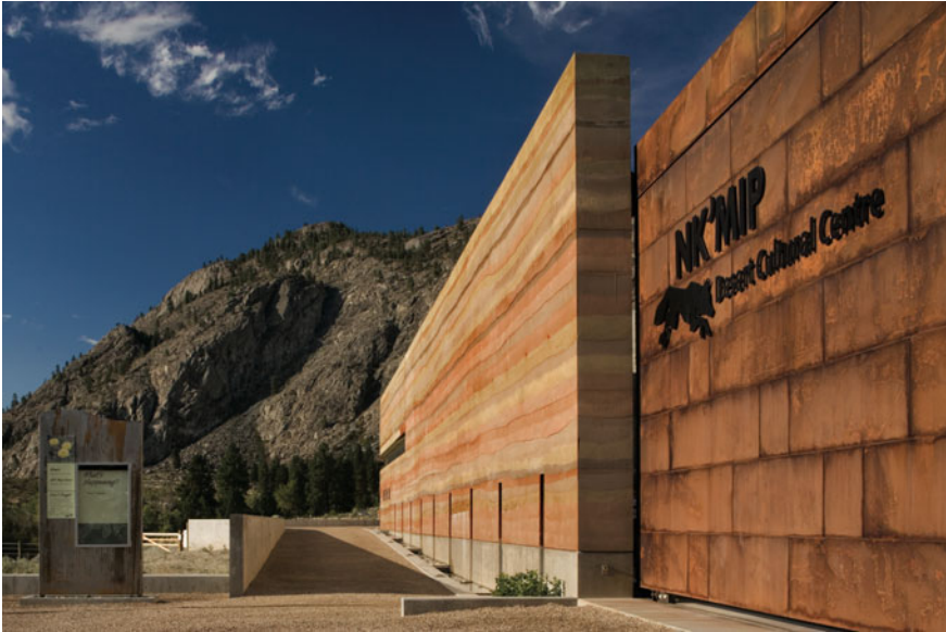
Fig. 8.1 Nk'Mip Cultural Centre (rammed earth wall) (Photograph Nic Lehoux)
