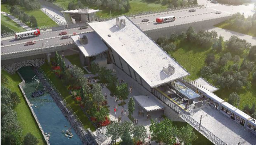
Fig. 9.4 Pimisi Station, confederation LRT Line, Ottawa ( Image City of Ottawa)
