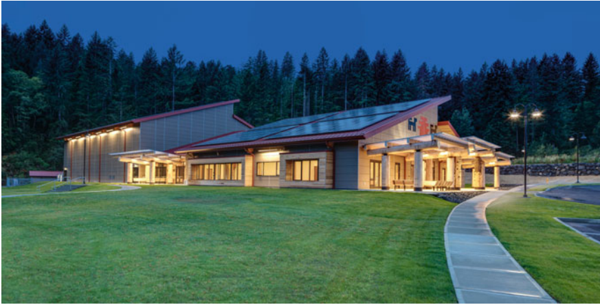
Fig. 28.10 Skokomish Community Center, 2017 ( Photograph Doug Walker, courtesy of 7 Directions Architects/Planners)
