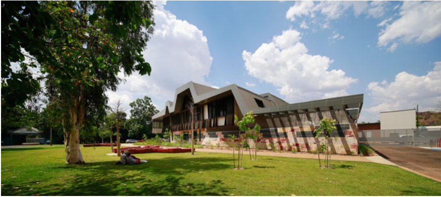
Fig. 19.10 Kununurra Courthouse exterior ( Photograph Peter Bennetts )
