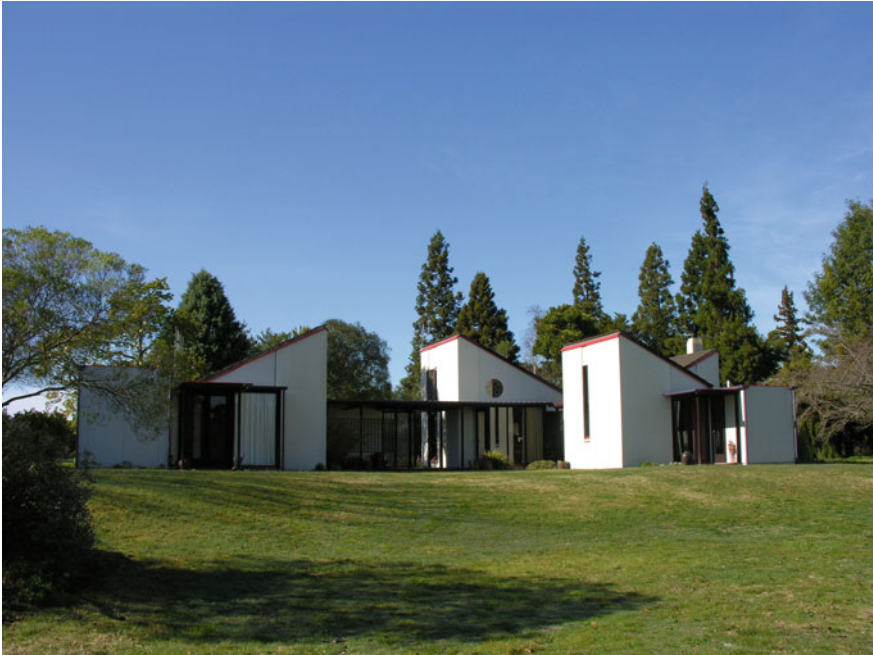
Fig. 23.10 The Martin House at Bridge Pā (1968–70), comprising a series of small pavilions (Photograph Julia Gatley)
