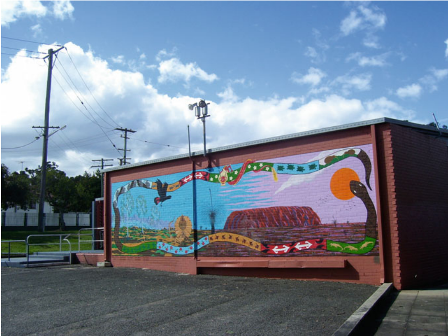
Fig. 20.7 The Old LibraryLibrary, Kev Hooper Park, Inala, featuring murals on all sides of the building, 2008 ( Photograph Kelly Greenop )
