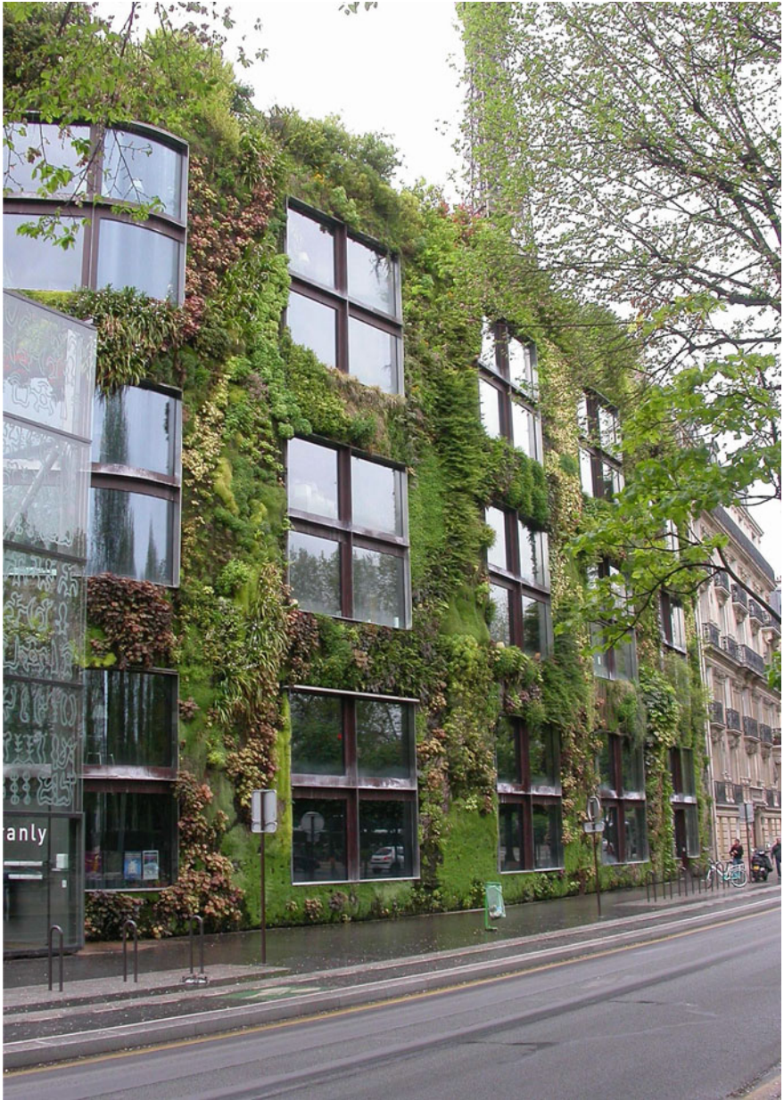
Fig. 34.7 Patrick Blanc-designed green wall on the quai Branly wing of the MQB; to the left is part of the glazed screen that encloses the museum's northern boundary ( Photograph Paul Walker )
