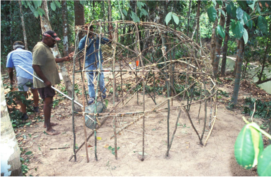
Fig. 16.8 Sapling and rattan lattice mija frame constructed by Girramay and Gulngay builders in 2004 ( Photograph Timothy O'Rourke)
