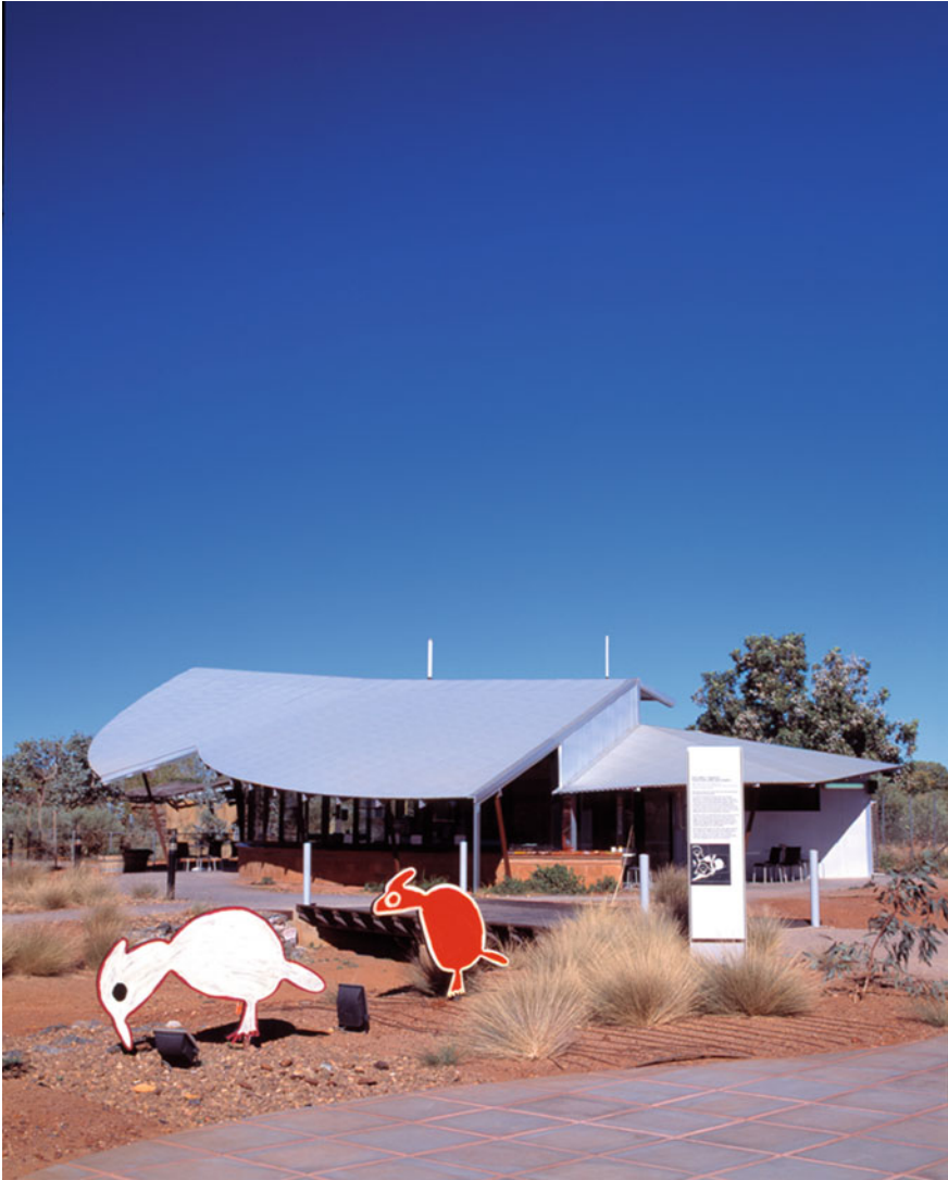
Fig. 15.2 Nyinkka Nyunyu Art and Culture Centre, Tennant Creek, Northern Territory ( Photograph Tangentyere Design)
