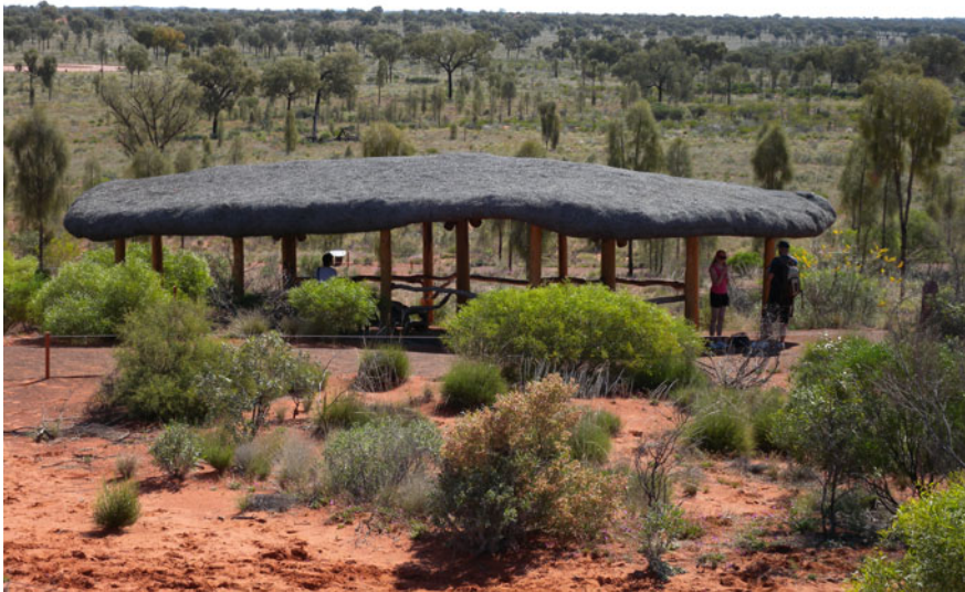
Fig. 16.10 Visitor shelters thatched with spinifex in the Uluru-Kata Tjuta National Park in Central Australia, 2010 (Photograph Rodger Barnes)
