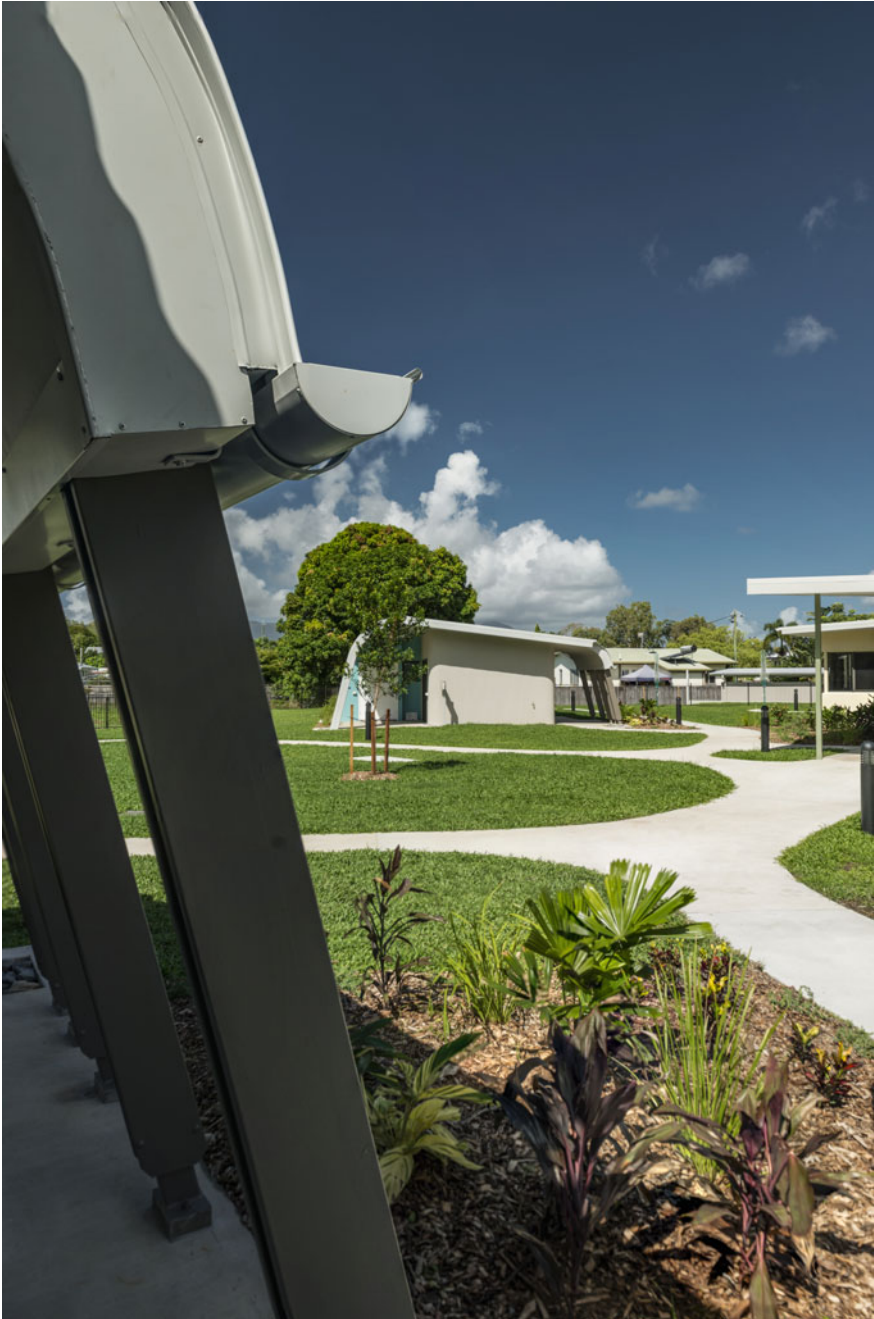
Fig. 17.7 Synapse SAIF, side view of accommodation units ( Photograph Michael Marzik )
