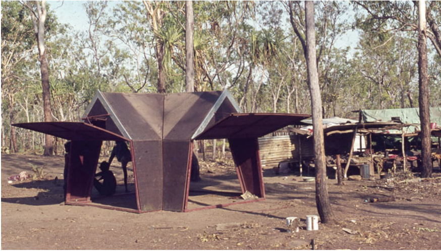
Fig. 2.4 Prefabricated Goorawin Shelter by Architect Ed Oribin for the ATSIHP at an outstation in Arnhem Land, 1977 ( Photograph Michael Heppell )
