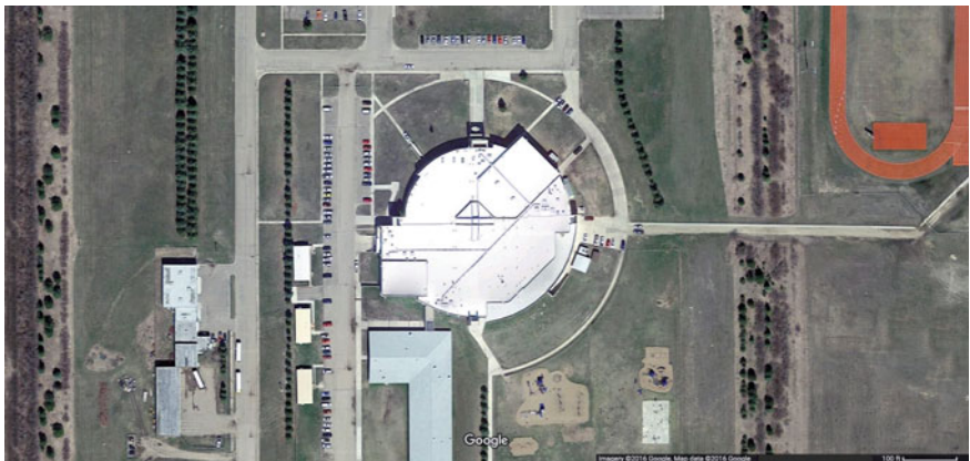
Fig. 6.4 Four Winds High School showing the circular shape ( Image Google Maps 2016)
