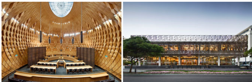
Fig. 19.1 The Supreme Court of New Zealand complex in Wellington, Aotearoa New Zealand. Warren and Mahoney Architects wrapped the building in a complex eight-metre-high bronze screen referencing Rata and Pohutukawa trees in a design strongly influenced by Māori concepts. In the centre of the building is the orb-shaped courtroom finished in panels of silver beech timber (Photographs Warren and Mahoney Architects)
