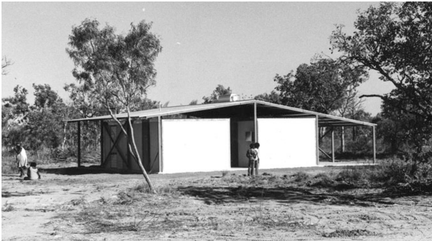
Fig. 2.5 One of John Flower's designs for housing in Mowanjum, Western Australia, for the Aboriginal Housing Panel, 1977 (Photograph Balwant Saini)
