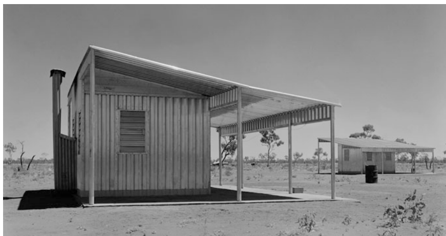
Fig. 2.3 Kingstrand houses at Warrabri Government Settlement, Northern Territory, 1958 (Photograph W Pedersen National Library of Australia)
