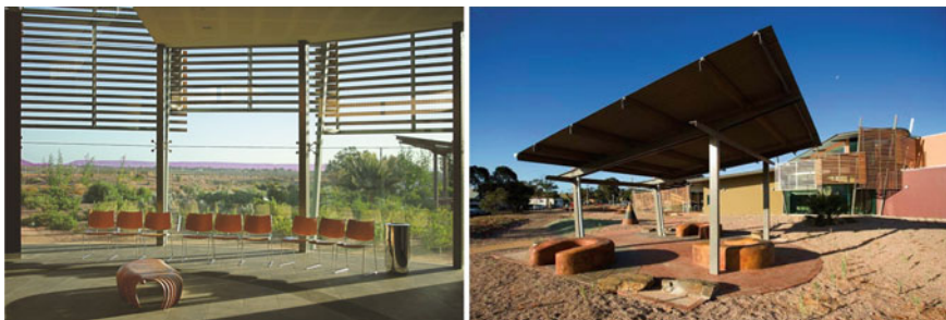
Fig. 19.5 Port Augusta Courthouse, internal and external waiting areas. The external waiting area has the capacity to function as an outdoor courtroom but has not been used for that purpose (Photographs Georgie Sharp)
