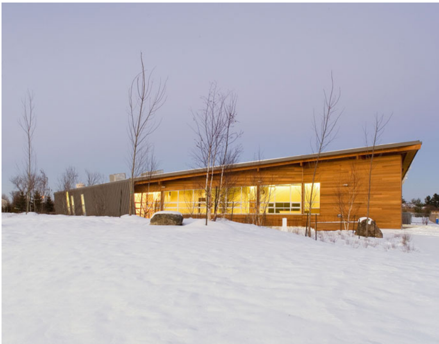
Fig. 33.4 Binoojiinsag Kinoomaagewgaming's roof rises from the earth towards the sun (Photograph Tom Arban Photography)
