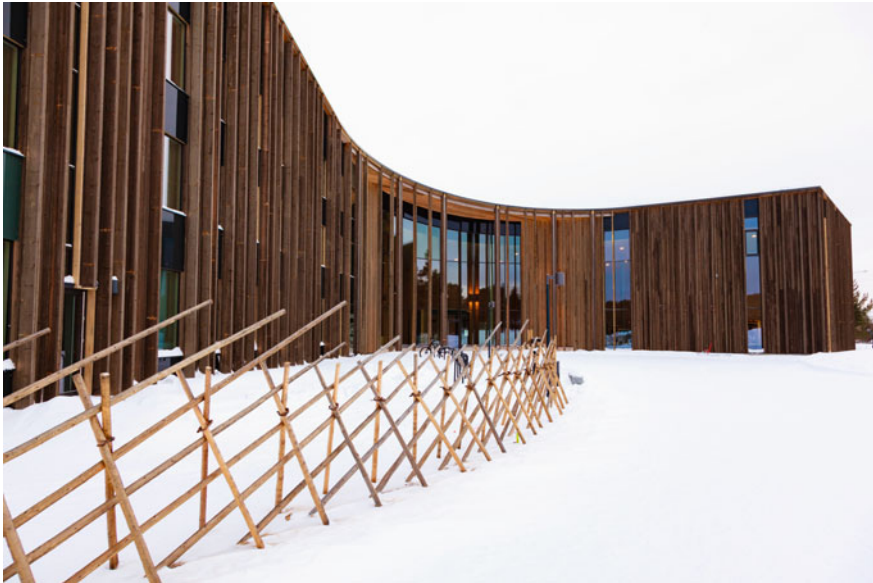
Fig. 30.8 Sajos in Inari, housing the Finnish Sámi Parliament and Sámi Cultural Centre. The construction is cast in situ concrete; the facade is made of full-height fir-tree planks treated with iron sulphates. Surrounding the curved walls of the building is a traditional type of fence which was used in this Sámi area. Sajos is designed by southern Finnish-based HALO architects, 2008–2012 (Photograph Anthony McEvoy)
