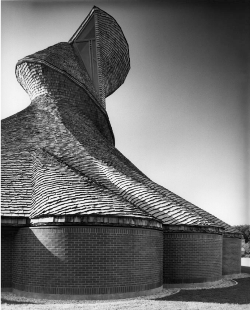
Fig. 10.8 Église du Précieux Sang/Precious Blood Church, Winnipeg. Designed by Étienne Gaboury ( Photograph Henry Kalen)
