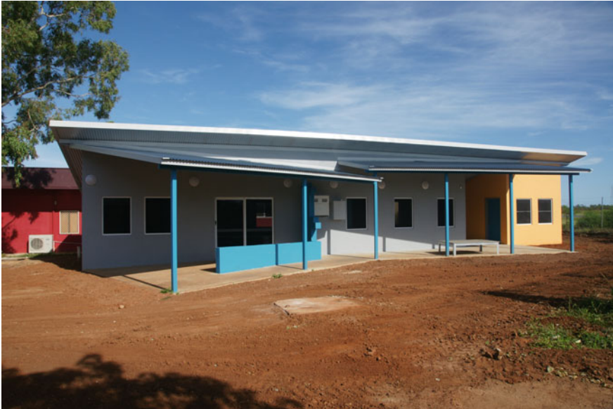
Fig. 13.5 Mornington Island Youth Media Building ( Photograph Indij Design)
