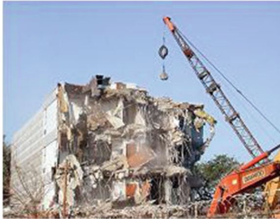
Fig. 2.2 Demolition by wrecking ball technique (Adopted from Prakash 2014)
