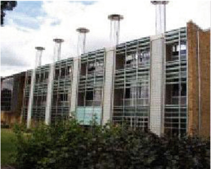
Fig. 1.5 The BRE office building in Watford, UK, 1995/96 (BRE 1998). For the foundations, a C25 mix (75 mm slump) was used with a minimum OPC-based cement content of 350 kg/m 3 and a maximum free water–cement ratio of 0.50 was required. For floor slabs, a C35 mix, also with 75 mm slump was specified. Over 1500 m 3 of RAC supplied for foundations, floor slabs, structural columns, and waffle floors
