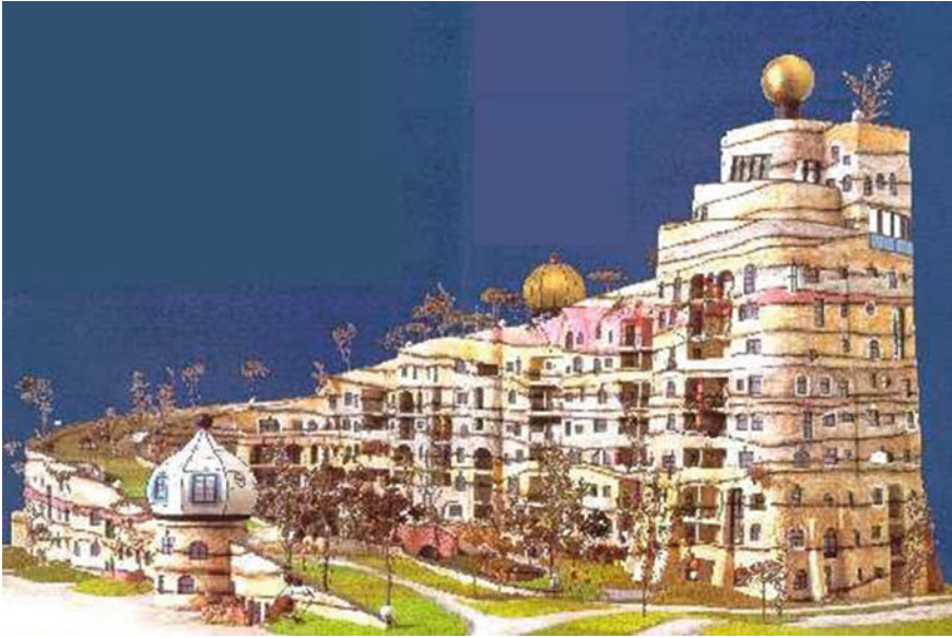
Fig. 1.6 Waldspirale residential building in Darmstadt, Germany, 1998 (Marinkovc and Ignjatovic 2010) Total 12 000 m 3 of RAC was built in (Source: http://www.b-i-m.de/projekte/projframe.htm )
