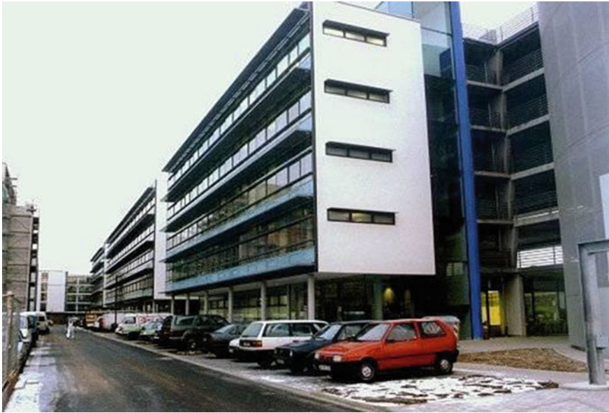
Fig. 1.7 Vilbeler Weg office building, Darmstadt, Germany, 1997/98 (Marinkovic and Ignjatovic Marinkovic and Ignjatovic 2010) Total 480 m 3 of RAC was built in (Source: http://www.b-i-m.de/projekte/projframe.htm )
