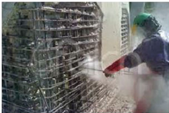
Fig. 2.5 Demolition by water jet (Prakash 2014)
