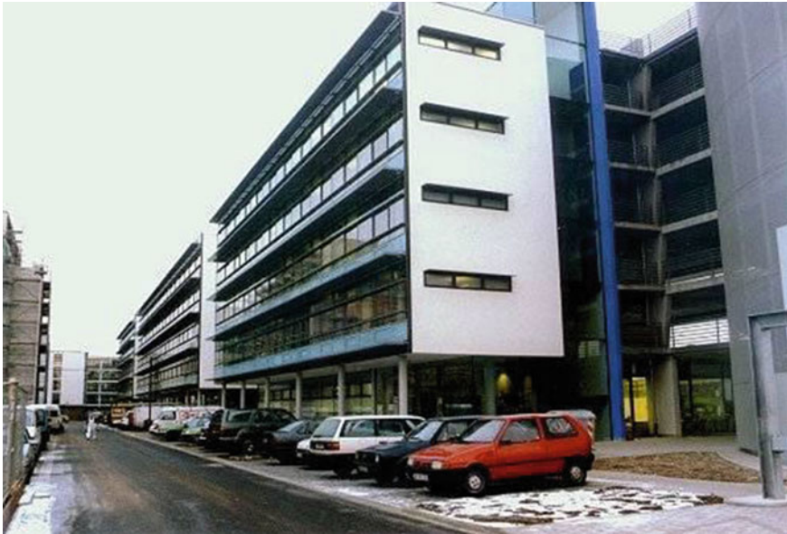
Fig. 1.7 Vilbeler Weg office building, Darmstadt, Germany, 1997/98 (Marinkovic and Ignjatovic Marinkovic and Ignjatovic 2010) Total 480 m 3 of RAC was built in (Source: http://www.b-i-m.de/projekte/projframe.htm )
