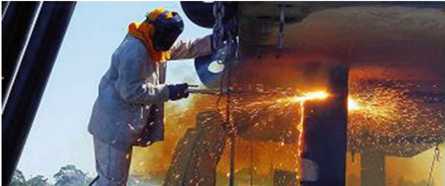
Fig. 2.4 Cutting of reinforcement through high temperature (Prakash 2014)
