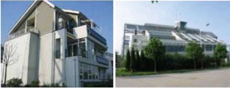
Fig. 1.4 Shanghai ecological building, China (Li 2008). This was a demonstrative ecological green building constructed in Xinzhuang, Shanghai, in 2004 with a total area of 1900 m 2 . Large amount of RAC (388 m 3 ) was used mainly in foundations and walls. The RCA was produced by crushing old concrete pavements and structural elements
