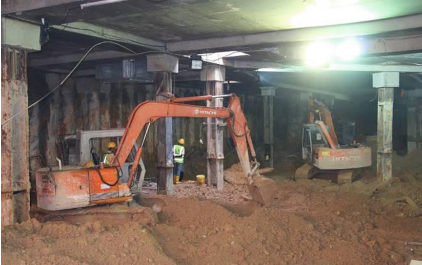
Fig. 6. Excavation works underneath the completed basement floor slab using top-down method
