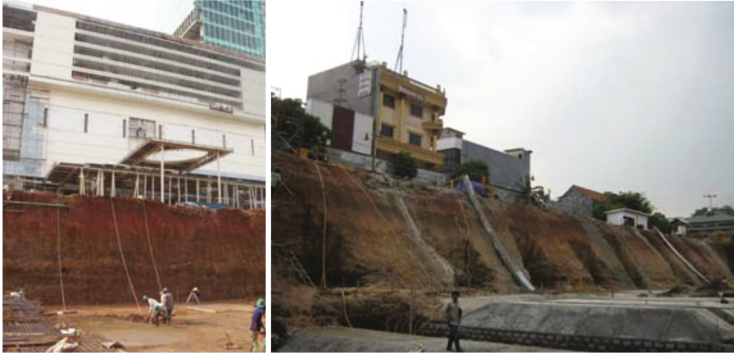
Fig. 6. Example of excavation at south of Jakarta with minimum protection
