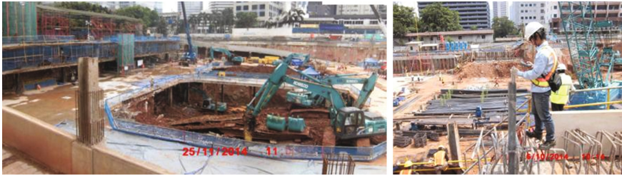
Fig. 25. Stage 2 excavation to 4th level Basement and measurement of D-wall movement
