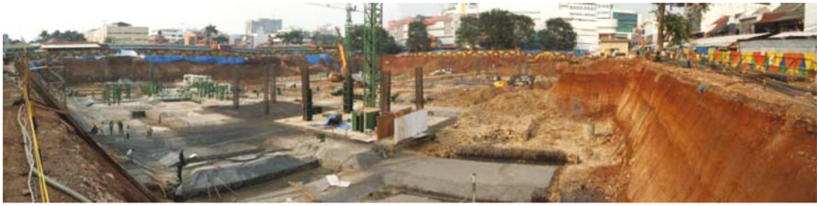
Fig. 7. Another example of 9 m depth of excavation at south of Jakarta
