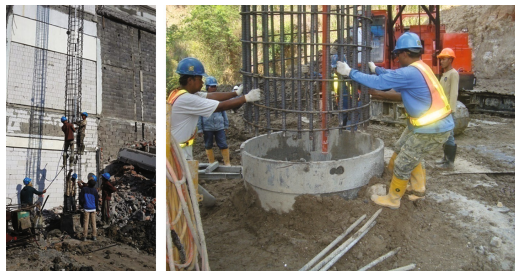
Fig. 12. Installation of inclinometers inside bored piles before excavation
