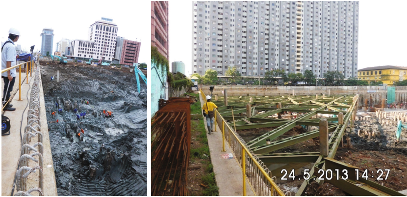
Fig. 31. Excavation in soft marine clays North Jakarta
