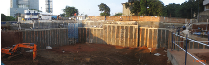
Fig. 14. Protection of excavation by soldier piles at South Jakarta
