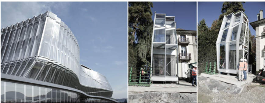
Fig. 1. Rendered output of the IOC façade ( left ). Mock-up of the final façade design ( right )
