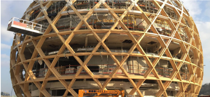
Fig. 1. The timber structure under construction
