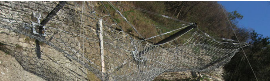
Fig. 2. Steel nets as rock fall barrier. © Maccaferri
