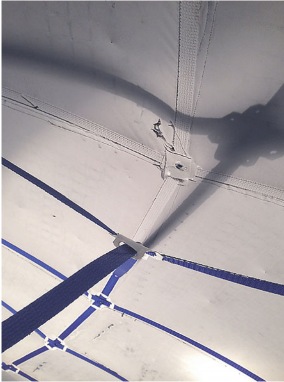
Fig. 18. Stripping the formwork, revealing the cast
