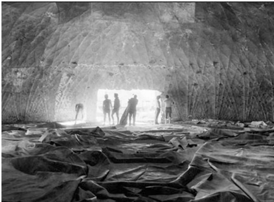
Fig. 2. Binishell, State Library of NSW, 1974
