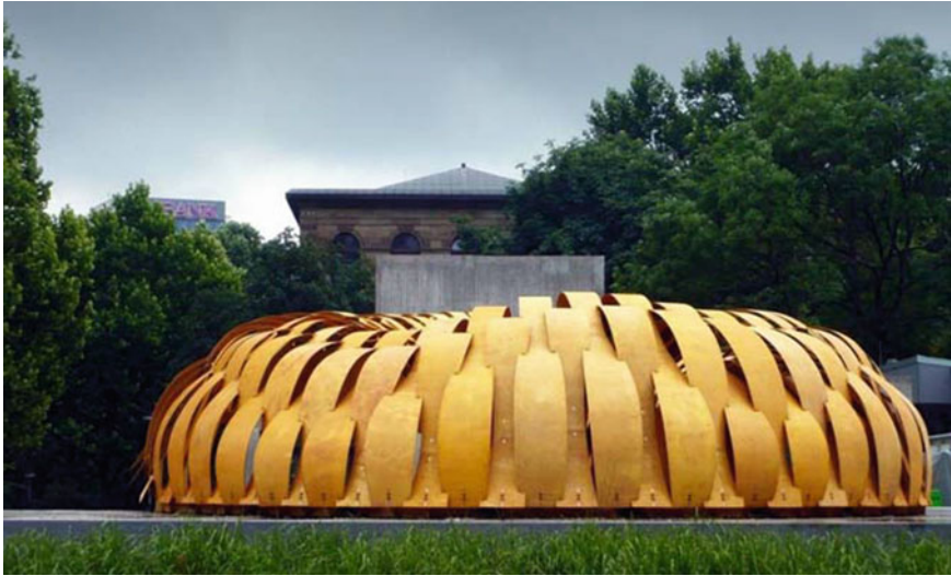
Fig. 1 Pavilion's envelope consists of wooden lamellas formed by an intricate network of bent and tensioned segments. This self-equilibrating system physically computes the shape of the pavilion during assembly on site. Institute for Computational Design (Achim Menges) and Institute of Building Structures and Structural Design (Jan Knippers), ICD/ITKE Research Pavilion 2010, University of Stuttgart, 2010
