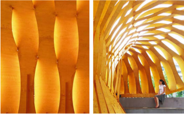
Fig. 2 Left The undulations of the thin wood lamellas, which are at the same time the pavilion's skin and structure, lead to differentiated direct and indirect illumination that accentuates the spatial depth. Right The residual stresses embedded in the building elements during assembly, which are a decisive factor in the structural capacity of the system, are experienced through the sinewy delicacy of the extremely thin wood lamellas
