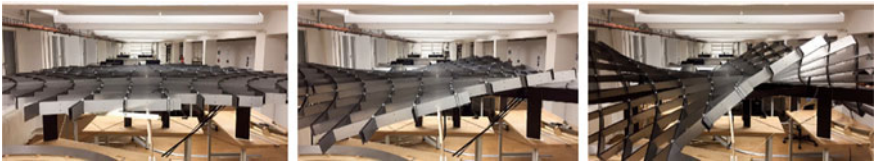
Fig. 12. Assembly process of the steel prototype, showing the elastic transformation from flat to curved geometry. Image Denis Hitrec
