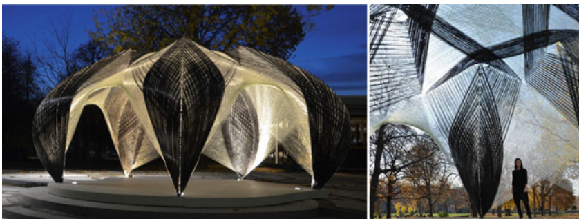
Fig. 3 Left The form of the pavilion’s composite shell gradually emerges through the interaction of fibres applied on a minimal scaffold during a robotic filament-winding process. Computation allows for understanding this complex material behavior in design and enables the strategic differentiation of fibre layout, organization, and density of fibres, resulting in novel fibrous tectonics. Right The pavilion’s skin structure is an extremely thin composite shell that does not require any additional support elements. In the translucent glass fibre surfaces, the black carbon rovings provide a distinctive visual reference to the intricate interplay between the fabrication- and force-driven fibre arrangements
