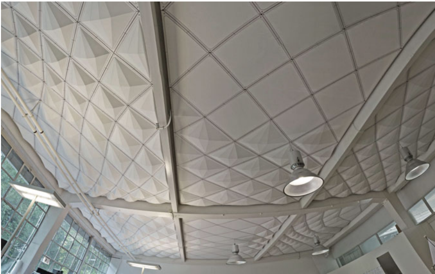
Fig. 1. Realized adapted acoustic ceiling composed out of self-similar elements—a typical property of digital process chains. Size and steepness of the modules express the proximity of sound emitting sources
