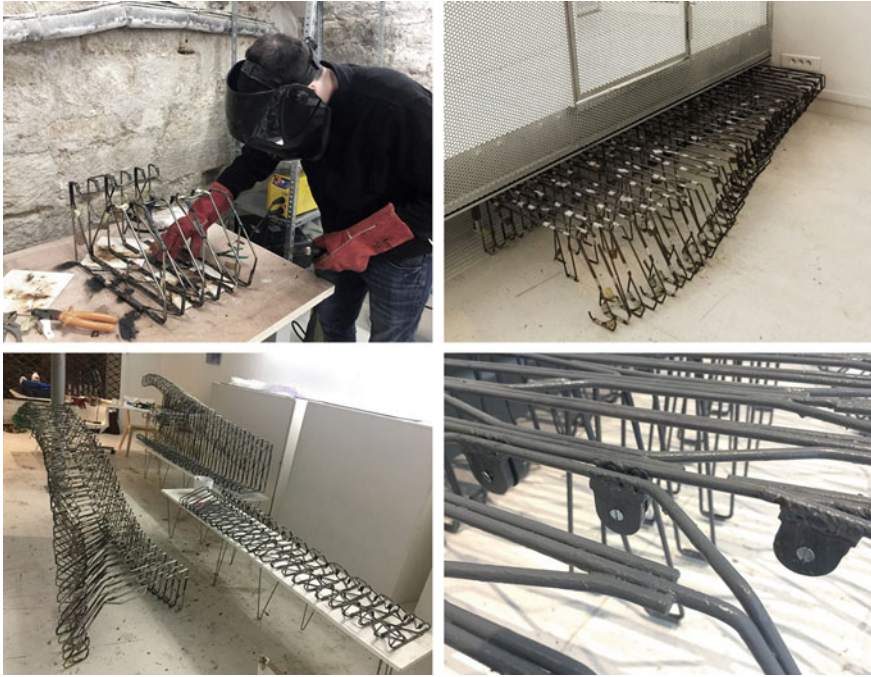
Fig. 13. Preassemble, welding, 3 final pieces and its joinery
