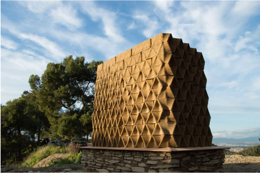
Fig. 8. Full scale prototype erected on site
