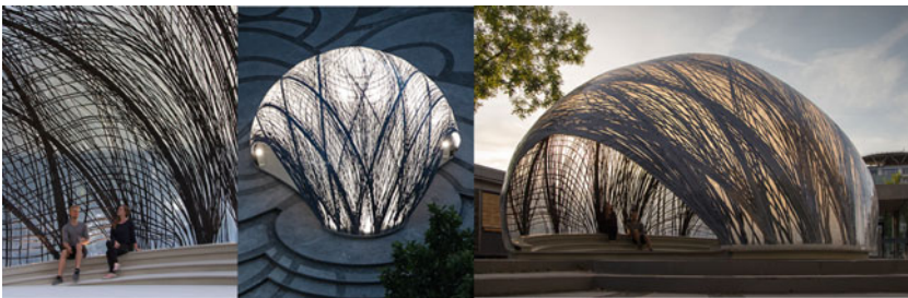
Fig. 4 Left The interior of the pavilion reveals the intricate carbon-fibre structure that articulates the spatial surface and at the same time provides the structural support for the transparent—and initially inflated—ETFE envelope. Center Computational design, simulation, and fabrication enable a synthesis of structure and skin that is perceived differently on the interior and exterior of the pavilion. During the day, only a subtle trace of the fibrous structure is visible on the reflective envelope, whereas the stark contrast between the transparent skin and the black carbon is strongly perceived on the inside. Right At night, the constructional logic of the cyber-physical design and fabrication approach remains tangible in the distinctive architectural articulation of the pavilion
