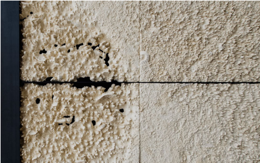
Fig. 9. Close-up of wall displaying the surface articulation resulting from a gradation of water pressure. ©ICD, K. Rinderspacher
