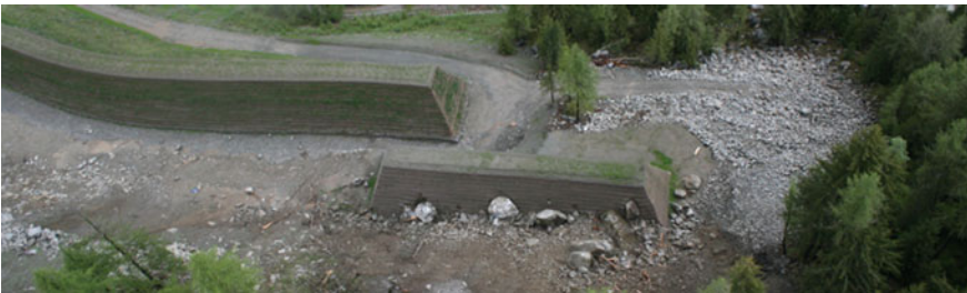
Fig. 3. Embankment used as rock fall energy dissipator. © Maccaferri
