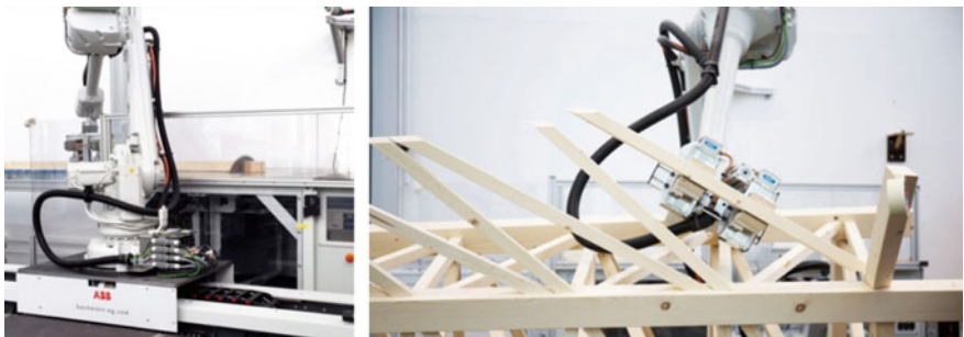
Fig. 7. Left Integrated saw cuts along robotic movements. Right Assembly of timber truss
