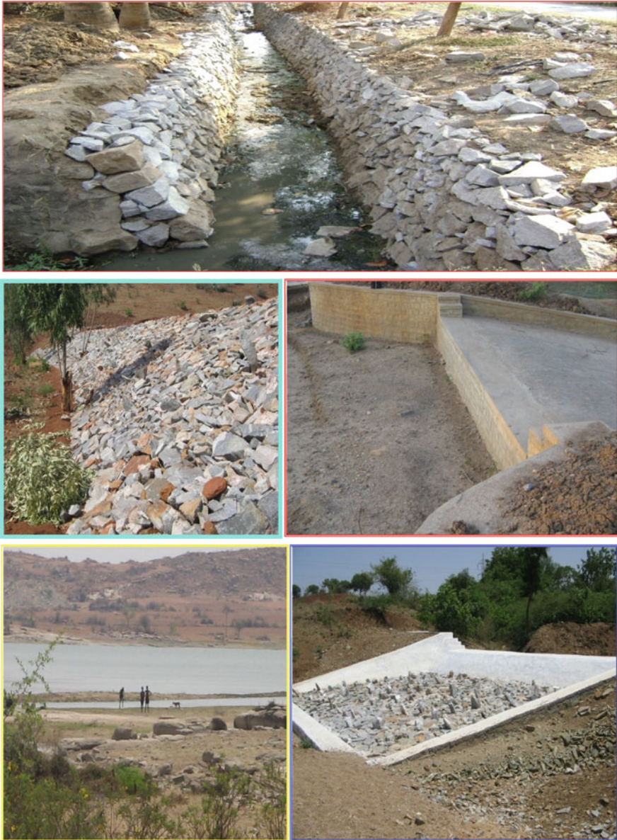
Fig. 11.4 Village development works taken up under MGNREGA
