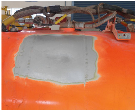
Fig. 14 Fuel tank after repair
