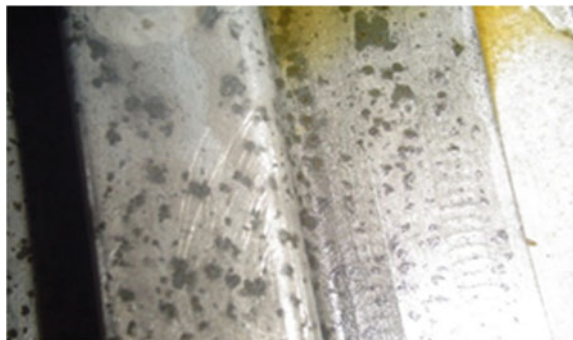
Fig. 5 Internal view of fuel tank showing pitting using endoscope/borescope
