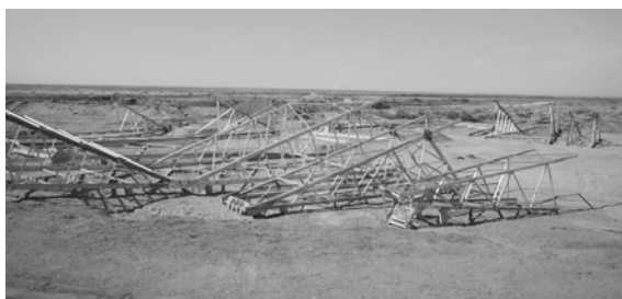
Fig. 4.25 Steel tower under construction (October 1, 2012)
