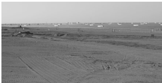
Fig. 4.24 Solar power plant, western suburb of Dunhuang (October 2, 2012)
