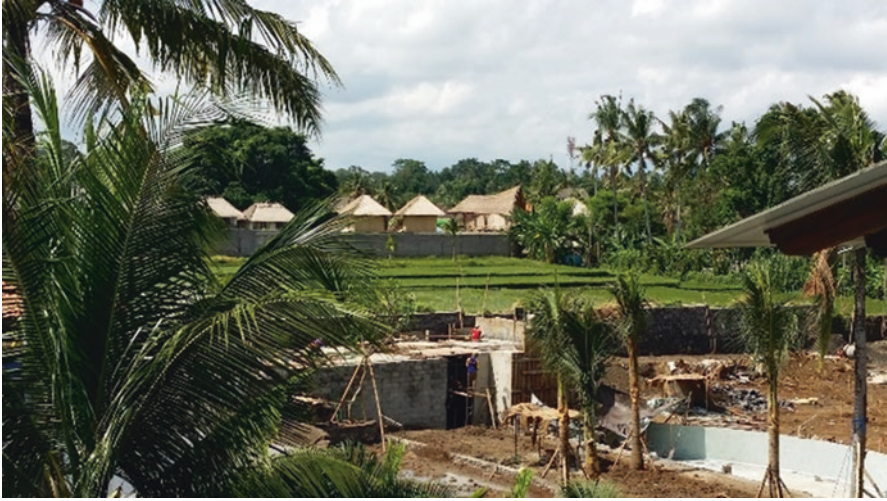
Fig. 7.2 Hotels under construction in rice fields, Ubud (Source: Author)
