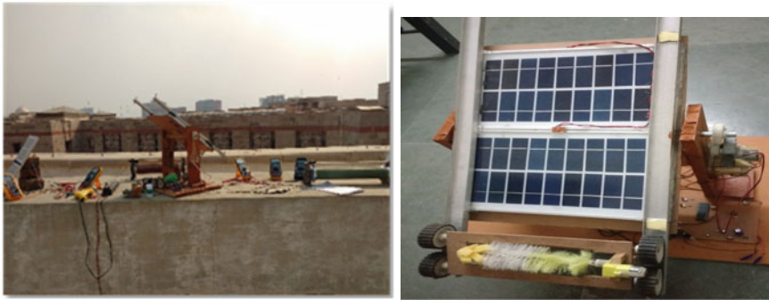
(a) Outdoor working of the Solar PV system (b) Close view of automatic cleaning PV system
