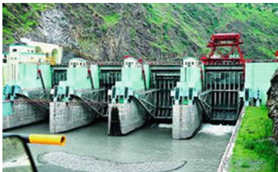
Fig. 2 Desilting chamber of Chamera-II
