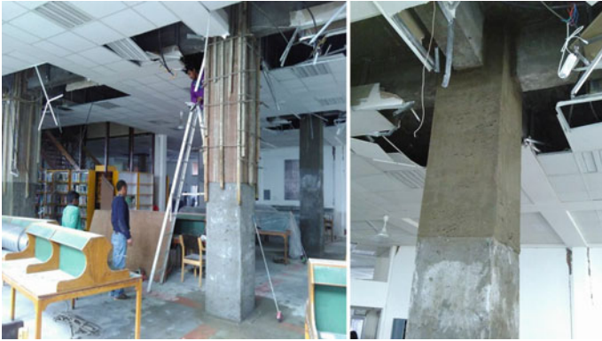
Fig. 7 Concrete jacking in columns of Kathmandu University Central Library (Dhulikhel)
