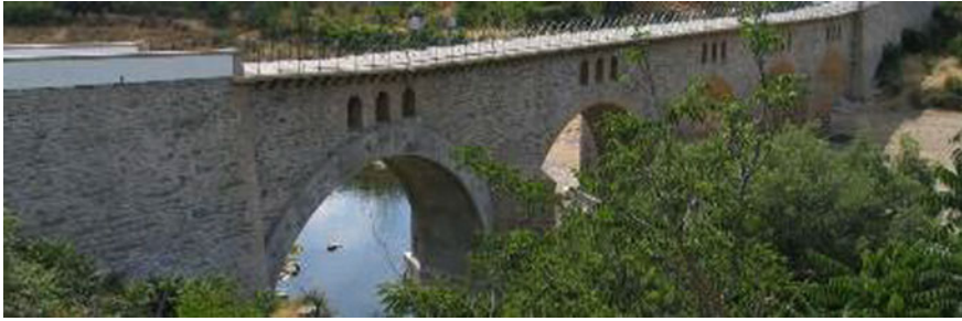
Fig. 12 Downstream view of Remondes bridge after the arch reinforcement with shotcrete
