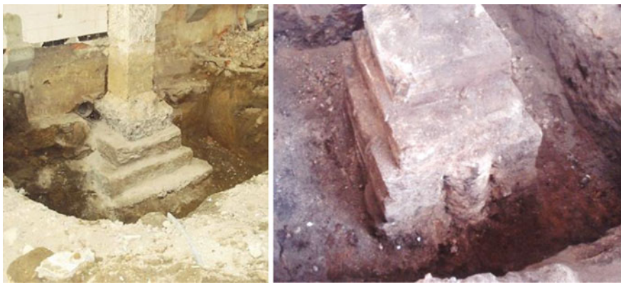
Fig. 28 Footing laying over a stone masonry, capping the original piles
