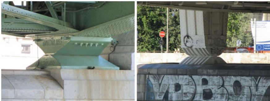
Fig. 14 Pin bearings in old steel bridges
