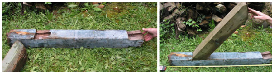
Fig. 1 Notched joints with tenons
