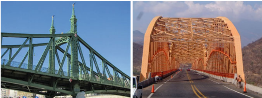
Fig. 2 Through-type truss bridges
