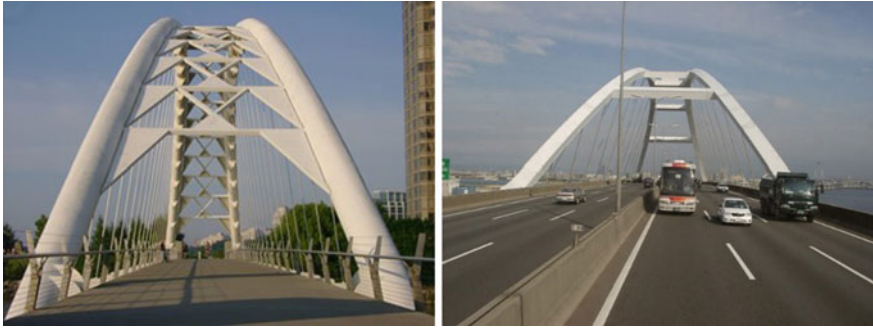
Fig. 5 Arch bridges with tubular- and box-type cross-sections
