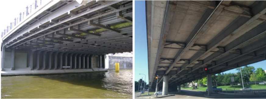
Fig. 8 Steel girder bridges
