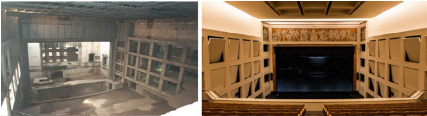
Fig. 12 Rivoli theatre building: view of the interior work already built
