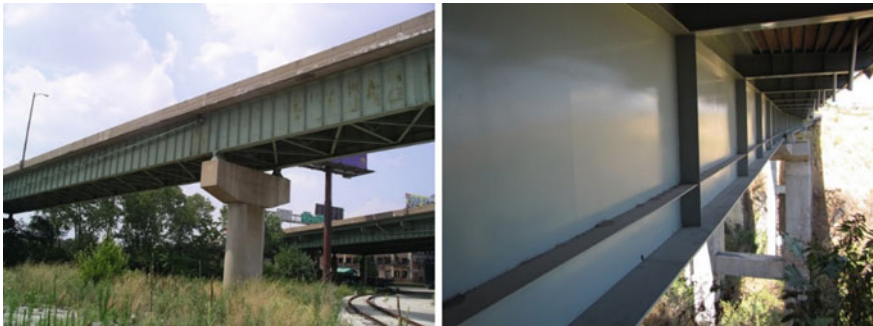
Fig. 9 Steel girder bridges with web stiffeners
