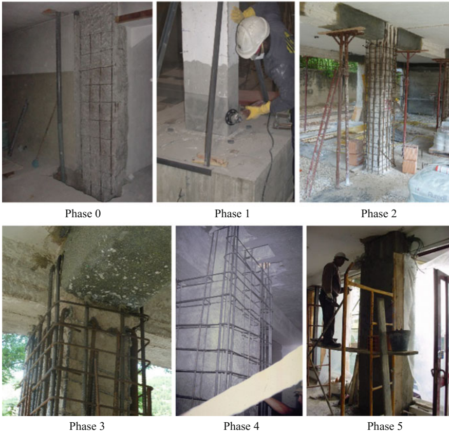
Fig. 1 Construction process of RC column jacketing
