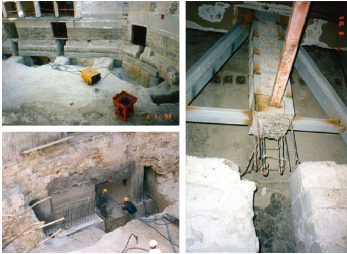
Fig. 11 Rivoli theatre building: execution of wells for underpinning
