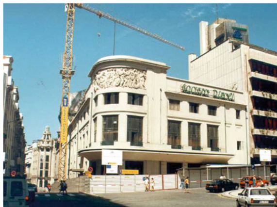
Fig. 4 Rivoli theatre building: external view when the rehabilitation started
