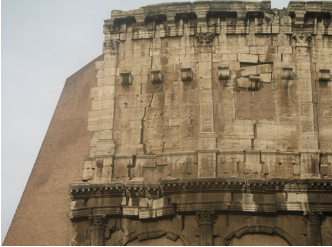
Fig. 2 Brickwork buttress of the Stern restoration (1807) of the Colosseum in Rome [7]
