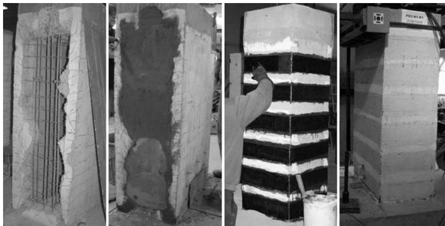
Fig. 3 Hollow piers before and after the shear retrofitting with CFRP sheets
