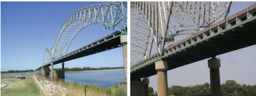
Fig. 6 Arch bridge with a truss structure
