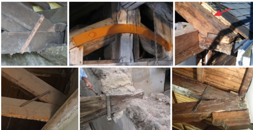
Fig. 8 Examples of original metal elements used in notched joints
