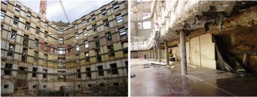
Fig. 1 Underpinning for the re-use of the façade of a building
