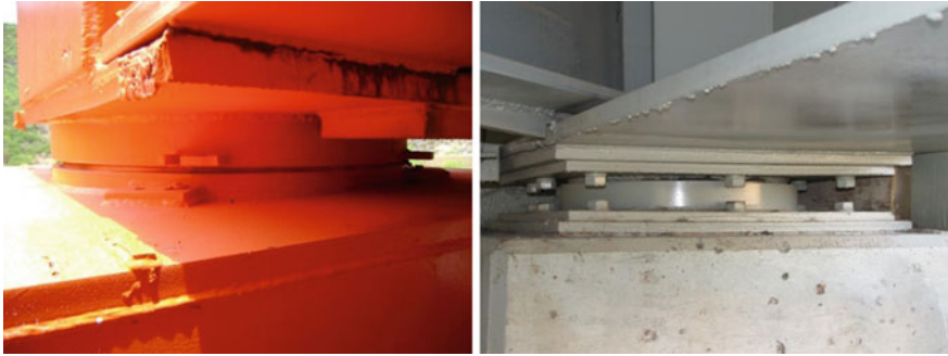
Fig. 16 Pot bearings in steel bridges
