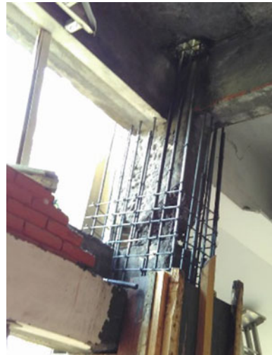
Fig. 7 Concrete jacking in columns of Kathmandu University Central Library (Dhulikhel)
