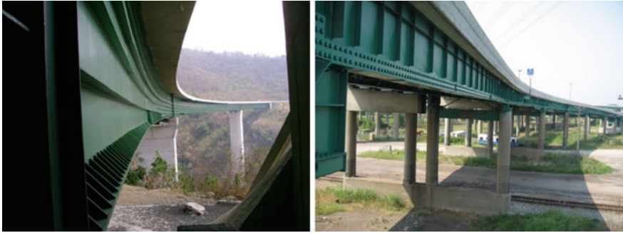
Fig. 13 Curved steel bridges
