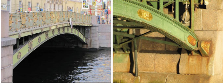
Fig. 3 Arch-type bridge with pin bearings
