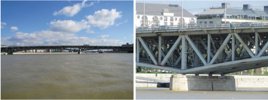
Fig. 1 Deck-type truss bridge
