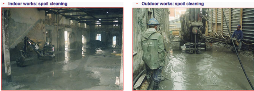
Fig. 22 Cleaning of the indoor and outdoor jet grouting spoil
