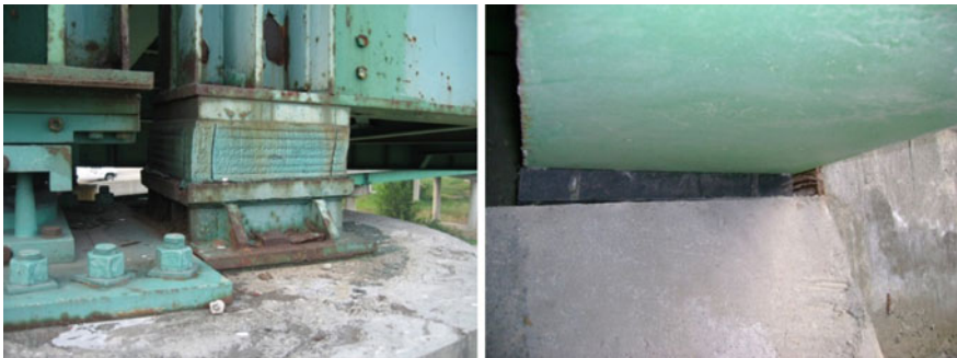
Fig. 15 Elastomeric bearings in steel bridges
