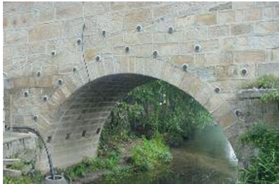
Fig. 19 Transverse ties in the bridge over the River Sul [46]
