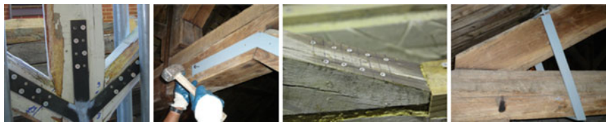
Fig. 9 Contemporary strengthening interventions on notched joints reproducing old techniques
