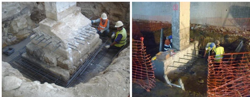
Fig. 29 Reinforcement of shallow foundations
