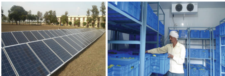
Fig. 3 A view of solar PV panel ( left ) and mango loading in the cold storage chamber ( right )
