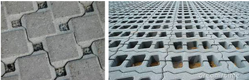
Fig. 5 Different arrangement of PICP pavements for parking. Image Courtesy google.co.in and perviousconcrete.org
