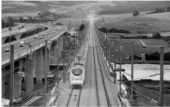
Fig. 4 A Eurostar train on Britain's first dedicated HS1 line linking London and the Channel Tunnel; note the smaller footprint compared with the parallel motorway
