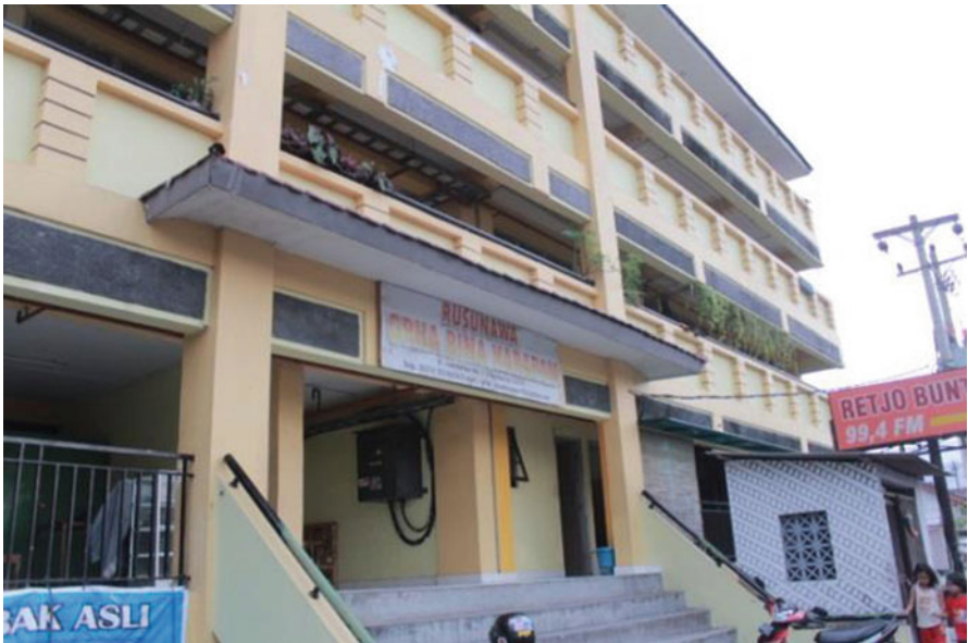
Fig. 15.6 Juminahan flats' front facade, Yogyakarta (Source: Author's Documentation, 2015)
