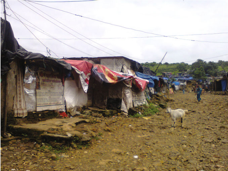
Fig. 14.1 Shanties and the temporary makeshift structures at Pimpripada. Source Authors
