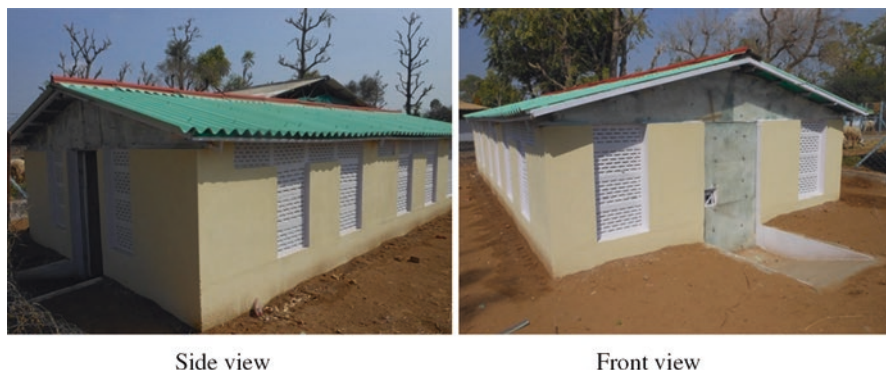
Fig. 16.2 Cold- and heat-protected thermocol-roofed shed for sheep
