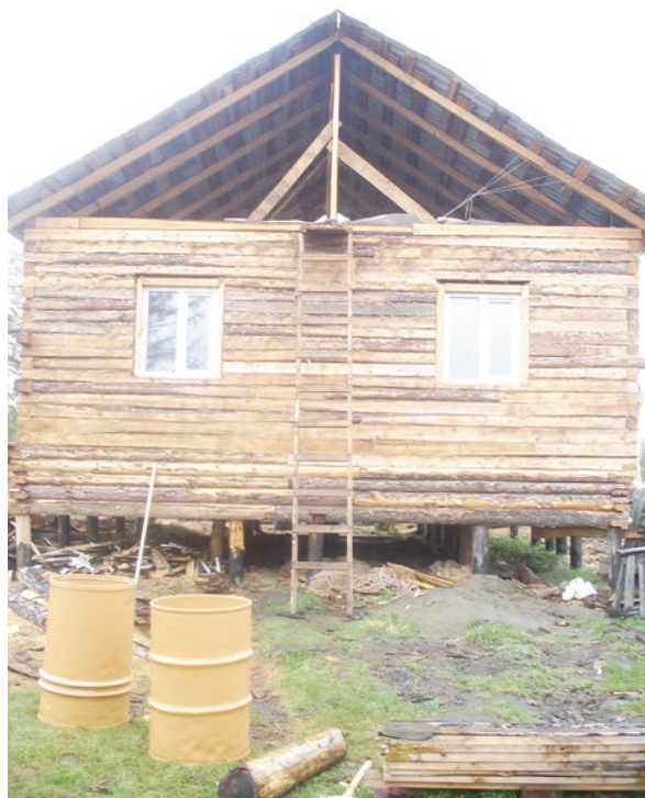
Fig. 2.8 The magnified image of the piles of house, an illustration of how villagers avoided the threat of floodwaters
