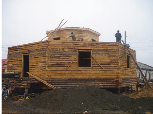
Fig. 2.9 Construction of the paleontological and ethnographic museum at Adycha secondary school, where the new timber is used for external look
