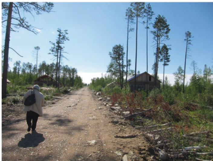
Fig. 8.6 Khatystyr: progress on construction of a new village (Photo by author)
