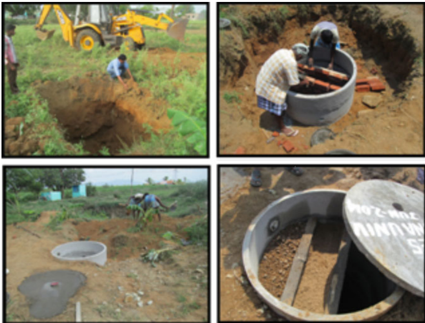
Fig. 6 Photographs taken during the construction
