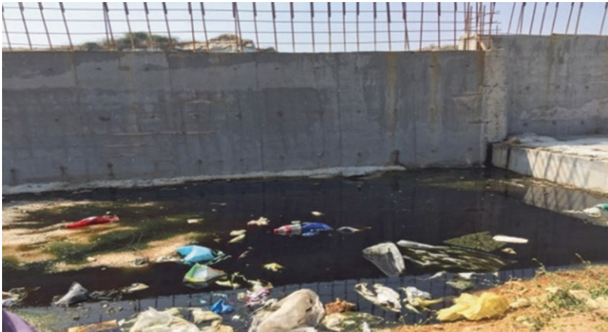
Fig. 21.6 Concrete wall for leachate containment
