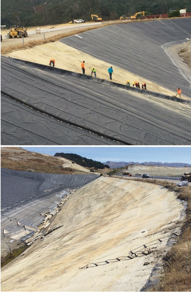
Fig. 23.2 Removal of liner system
