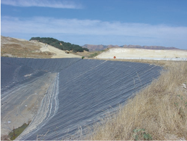
Fig. 23.1 Exposed liner system
