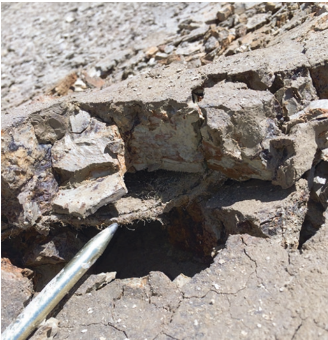
Fig. 23.6 Thickness of accumulated bentonite near toe of slope
