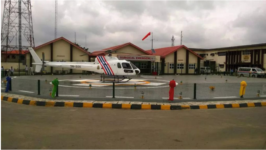
Fig. 2.5 Medical Helipad at the Lagos State University Teaching Hospital (LASUTH), Ikeja, Lagos. Source [24]
