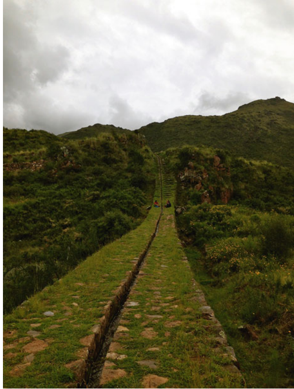
Photo 4 Inca hydraulic engineering work of Tipón (Image by Elizabeth Sumida Huaman)
