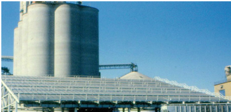
Fig. 8 A large-scale forced convection solar dryer
