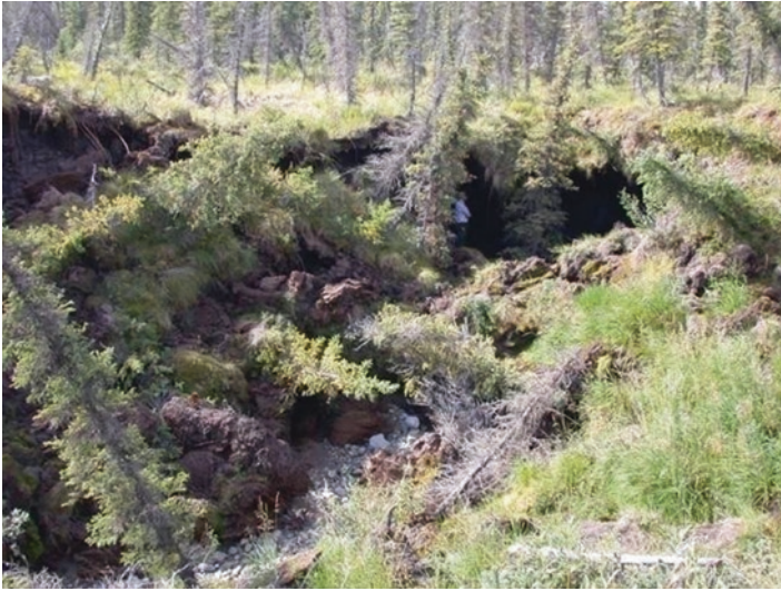
Fig. 22.7 Photo of ground collapse in the Noatak National Preserve in Alaska shows the thawing of permafrost as the climate getting warmer (Resource from Edward Schuur, University of Florida)
