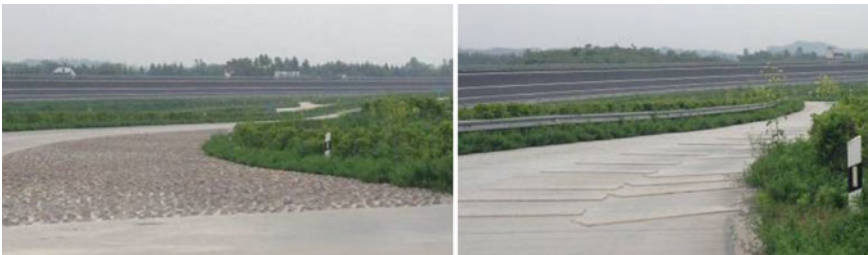
Fig. 44.1 Enhanced test roads on the proving ground
