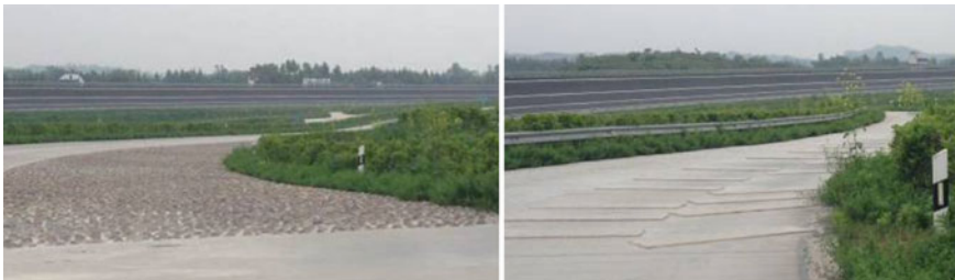
Fig. 44.1 Enhanced test roads on the proving ground
