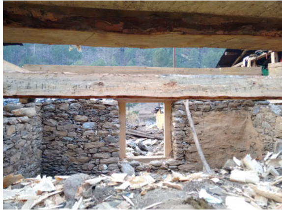
Fig. 8 On-going contemporary construction in typical Koti banal style of architecture in village Purola
