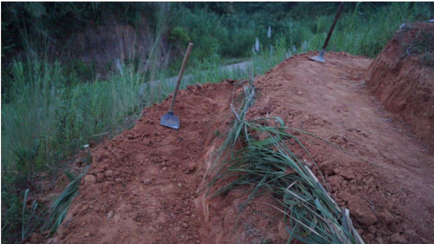
Fig. 6 Terraces formed with standard and modified spades
