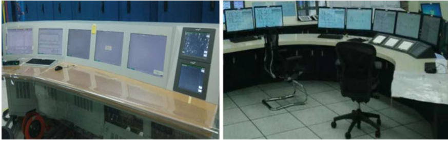
Fig. 5 Covered-type and bracket-type operator workstation
