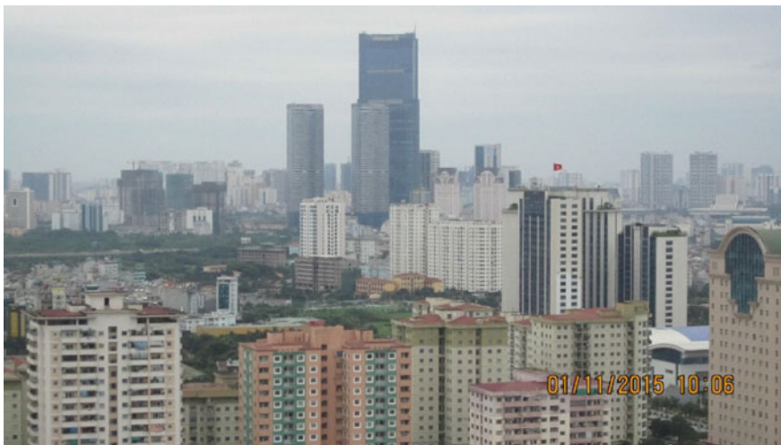
Fig. 7.2 A view of a highly urbanized area in Tuliem district, Hanoi City. Source Author’s fieldwork (2015)
