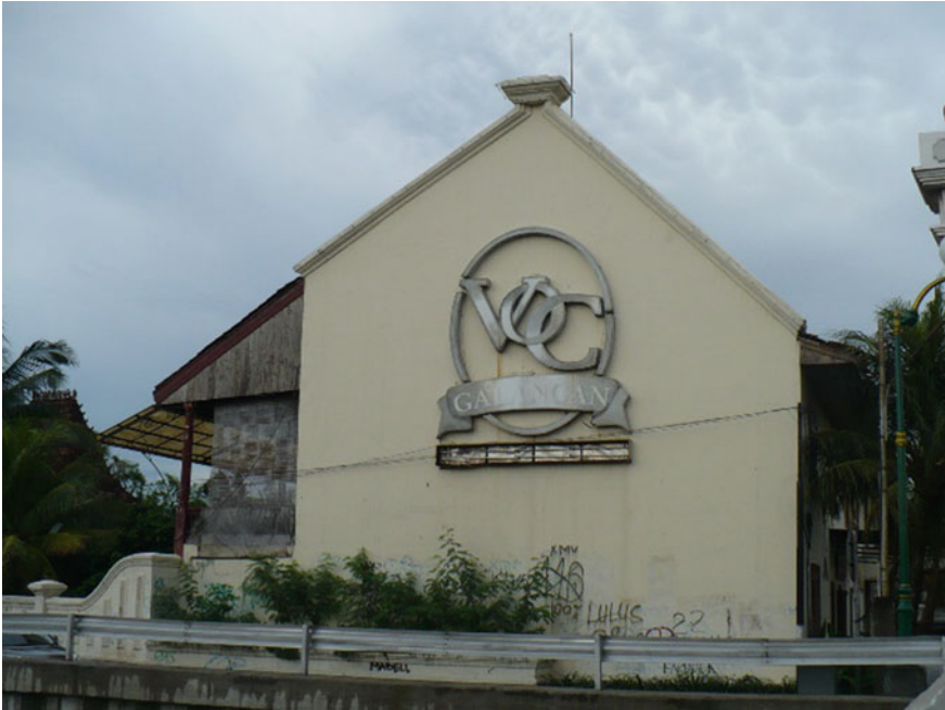
Fig. 6.3 A former warehouse of the Dutch East India Company. Source Author's fieldwork (2010)
